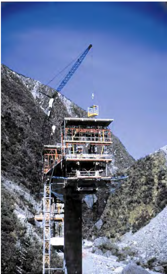
Oira Viaduct under construction
